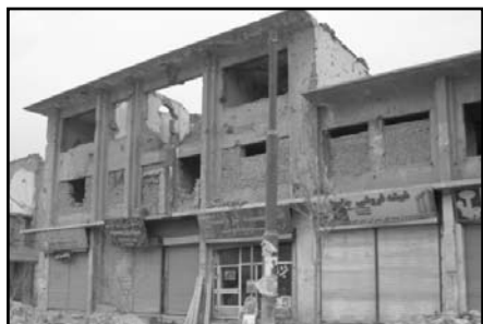
A typical scene of a battered house
